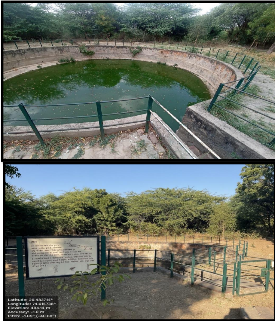
Fig 3.4: Rainwater Harvesting at RIE Campus
