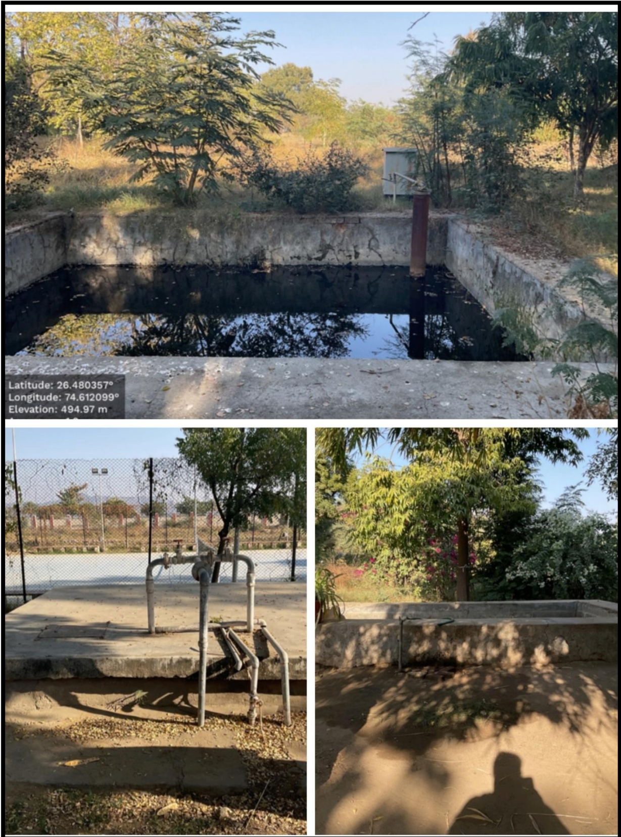
Fig 3.5: Water Tanks of RIE
